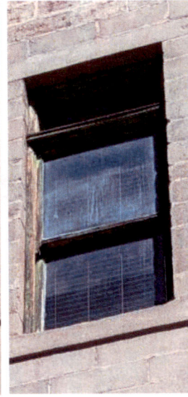
3 rd level wood windows in poor condition
