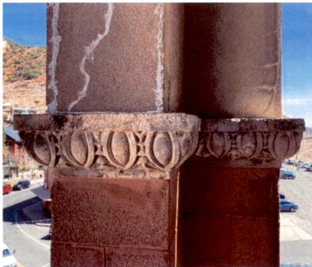
Delamination of unprotected exterior walls
