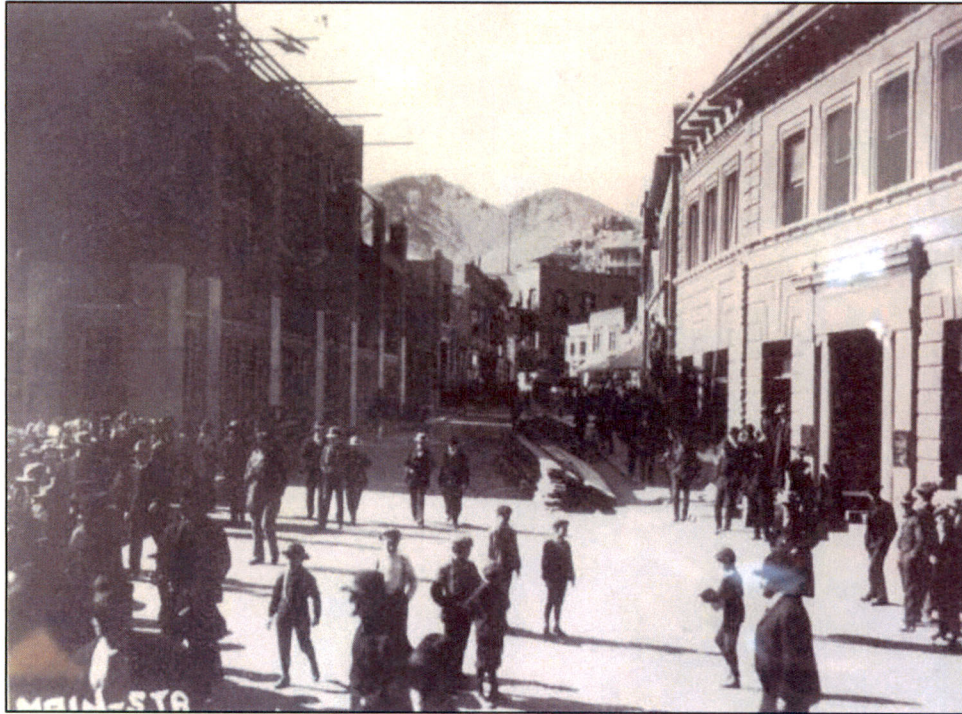
Figure 51. Main Street during construction, looking northwest. 1906. Courtesy of the City of Bisbee.
