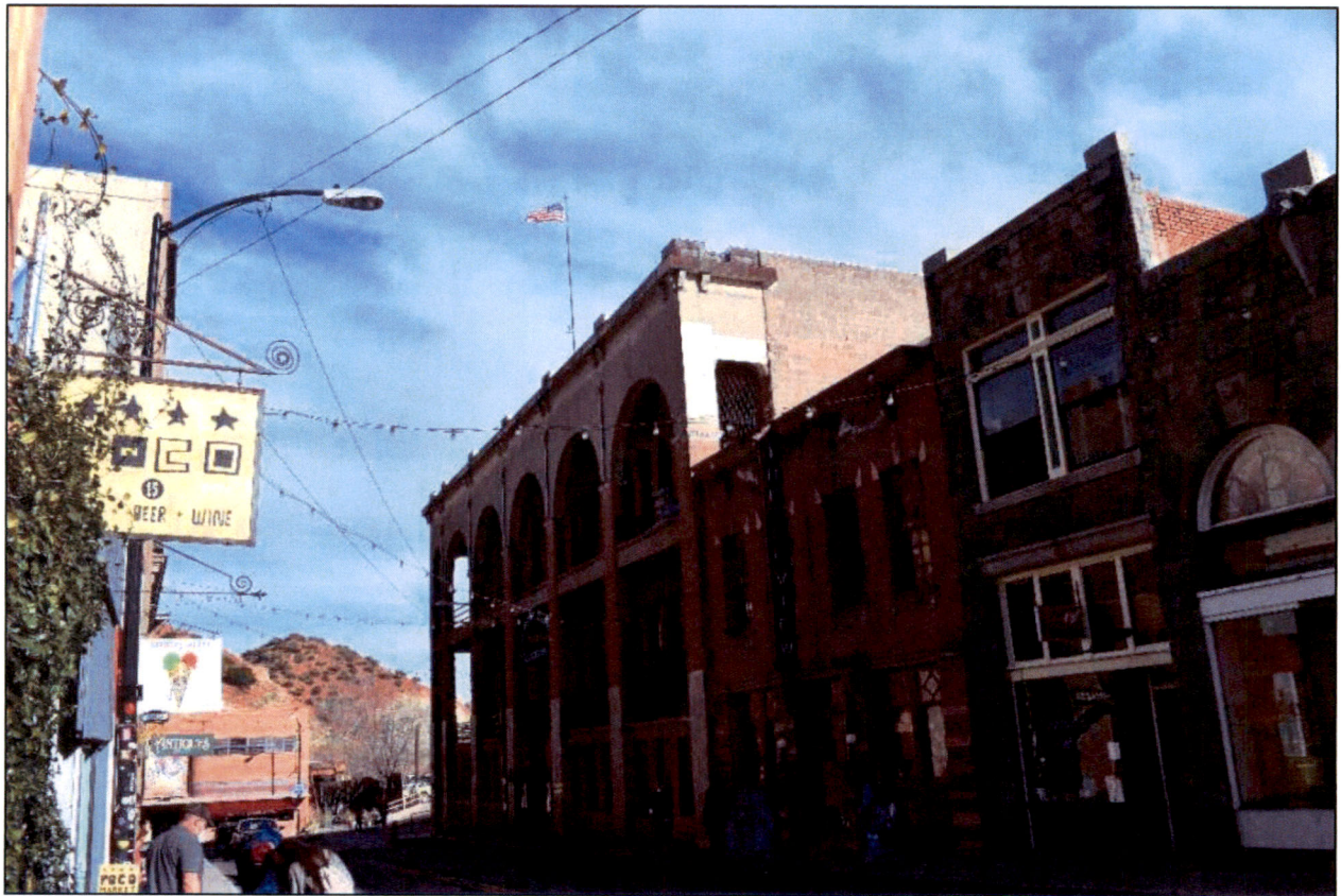
Figure 41. View of Copper Queen Library showing north and west elevations, looking southeast. Note the building's boxy form in the context of the street, its flush walls with the street edge and adjacent property, its perpendicular sides, and its flat roof. March 2021.
