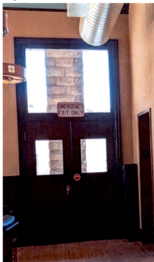
East exterior door to veranda (interior view)
