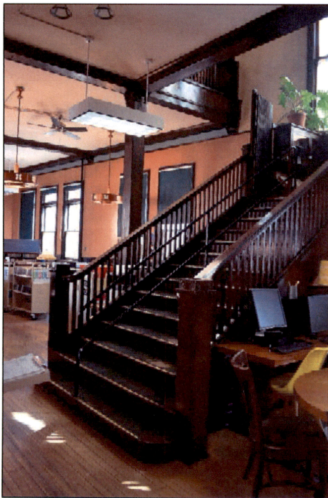
Figure 35. View of newel post, balustrade, stair treads, and risers. March 2021.
