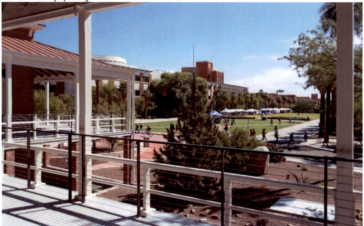
Old Main new safety railing
