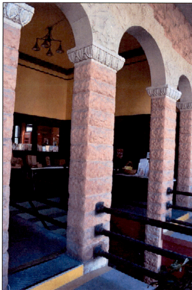
Figure 17. Library entrance vestibule in north elevation. March 2021.
