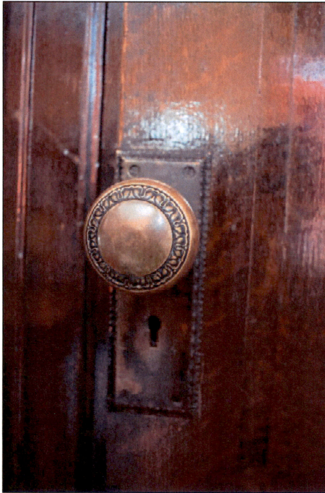
Figure 48. Doorknob on second story door beneath stairway. Small-scale features such as door hardware should, where possible, be retained and preserved. March 2021.
