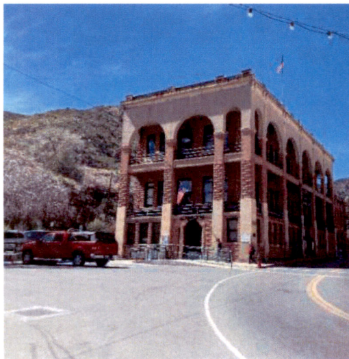
East parking area.
