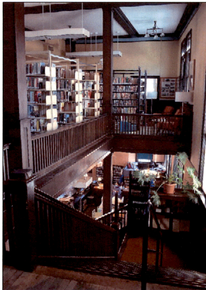
Figure 46. View of main stairway looking down from third story. The L-shaped circulation pattern of this stairway including its banister, woodwork, and lower gate should be preserved. Later elements including the metal hand rail or particle board flooring are not character-defining and may be removed or altered. Note that although these features are not representative of the building's original architecture, they are illustrative of its history and age and could be retained as a testament to the library's long-standing use. Library Bureau issued tables and chairs are original to building and should be preserved and retained. View looking east. March 2021.
