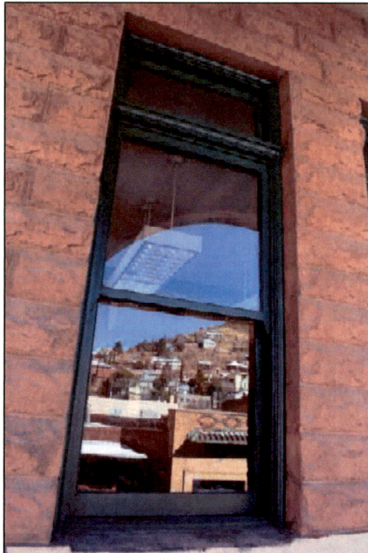
Figure 45. View of window along third story veranda of north elevation showing sash horns and ovolo molding. March 2021.
