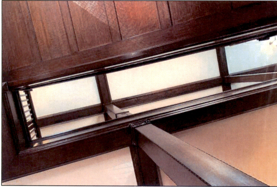
Figure 32. View of woodwork on wood-clad post adjacent to staircase showing box beams, ornamental beading, and capital. March 2021.
