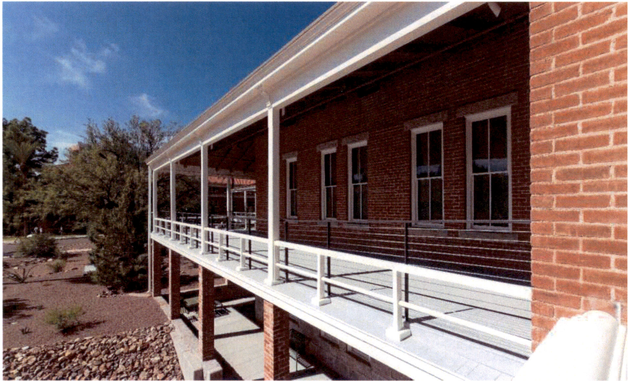
Old Main new safety railing
