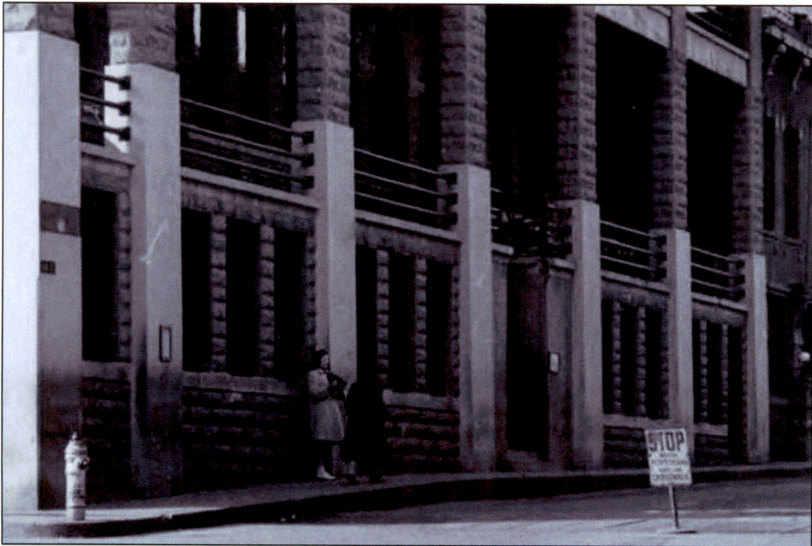
Figure 18. North elevation showing original configuration door at far right and without gate or signage. Circa 1940. Courtesy of the Pomona Public Library.
