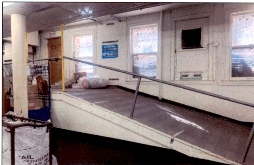
Figure 29. Post office sorting room ramp against south wall, looking south. March 2021.
