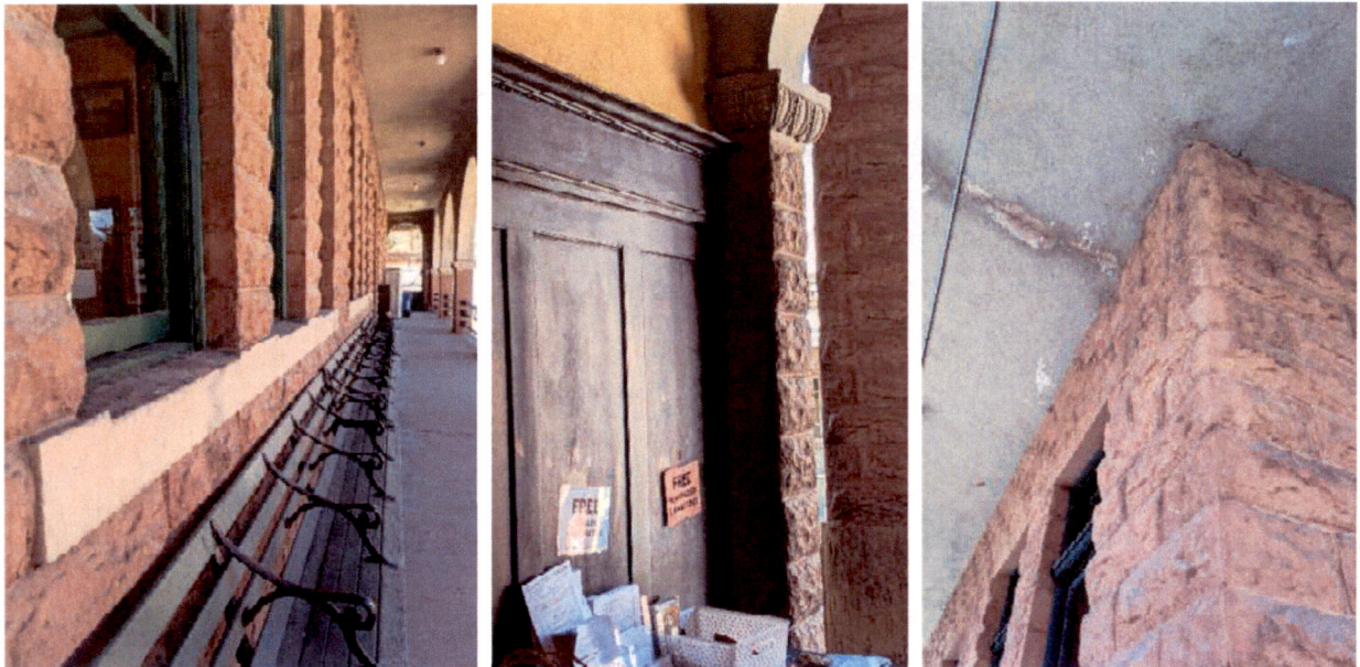
Protected exterior walls
