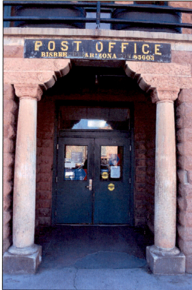
Figure 10. Recessed entry in east elevation of the Copper Queen Library. March 2021.
