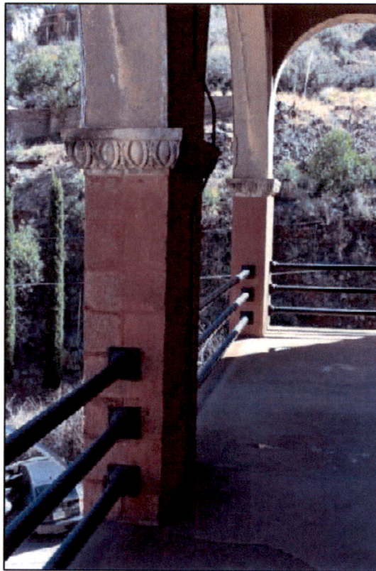
Figure 13. Third story veranda along east elevation showing arcade and railings. Looking south. March 2021.
