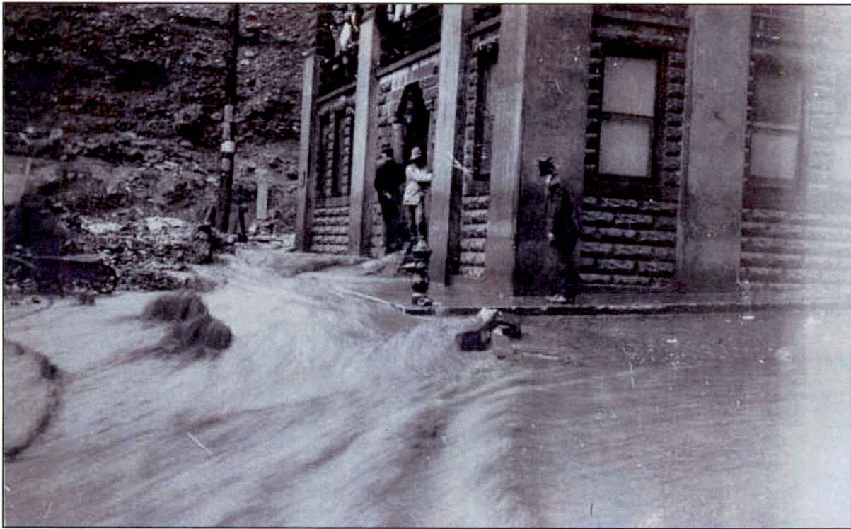
Figure 54. Photograph of debris around the Copper Queen Library after a flood, looking southwest. 1908. Courtesy of the City of Bisbee.
