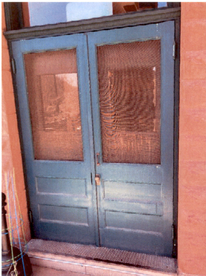
East exterior door to veranda (veranda view)
