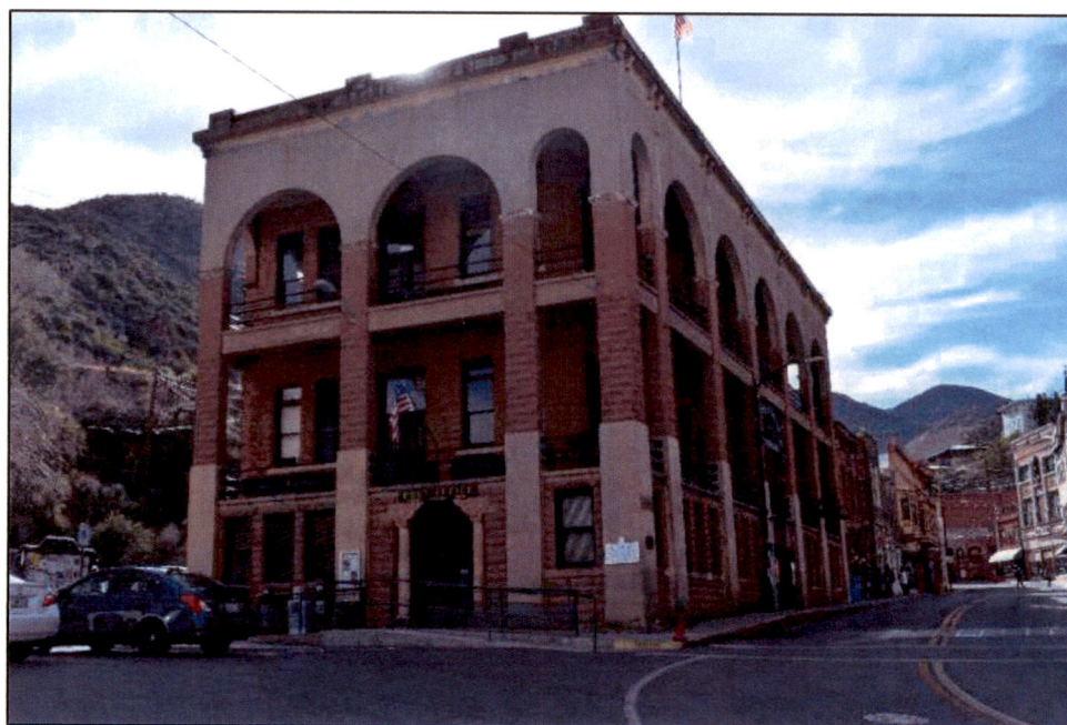
Figure 9. East elevation of the Copper Queen Library. March 2021.
