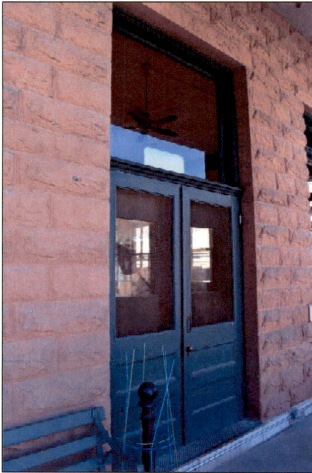
Figure 11. Exterior door in second story of east elevation. March 2021.
