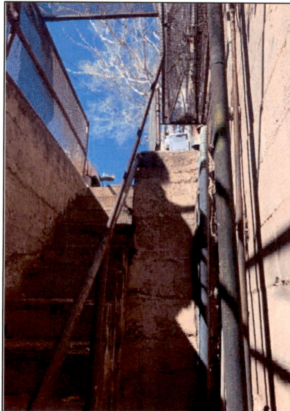
Figure 25. Access stair to partial basement, looking west. March 2021.
