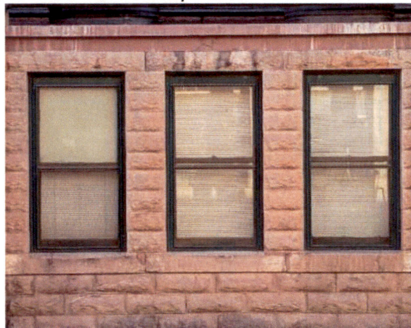
North windows facing Main
