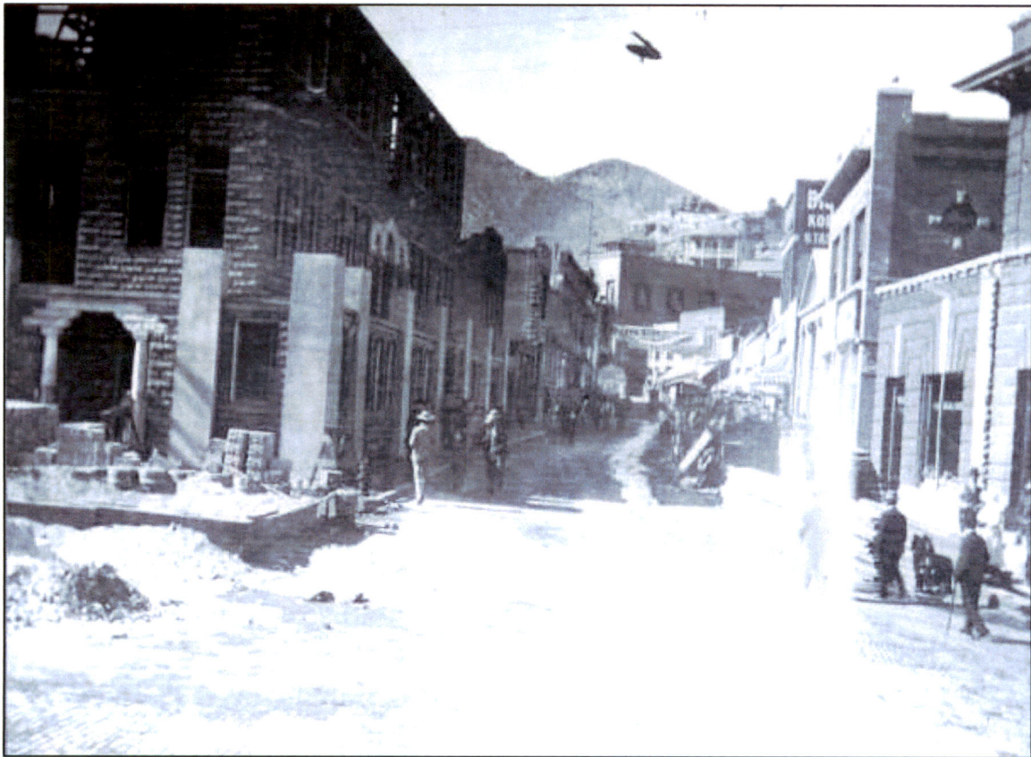
Figure 52. Stone block staging process during construction. 1906b. Courtesy of Copper Queen Library archives.
