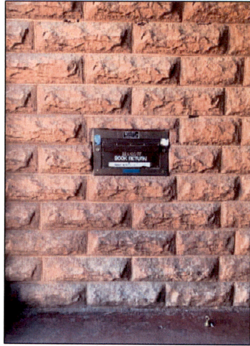
Figure 5. Rusticated light brown blocks within the recessed entry on the east elevation. March 2021.
