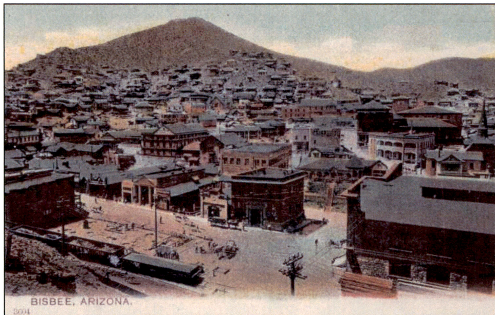
Figure 53. Postcard showing the foundations of the new building in the lower left corner. 1906a Courtesy of Copper Queen Library archives.
