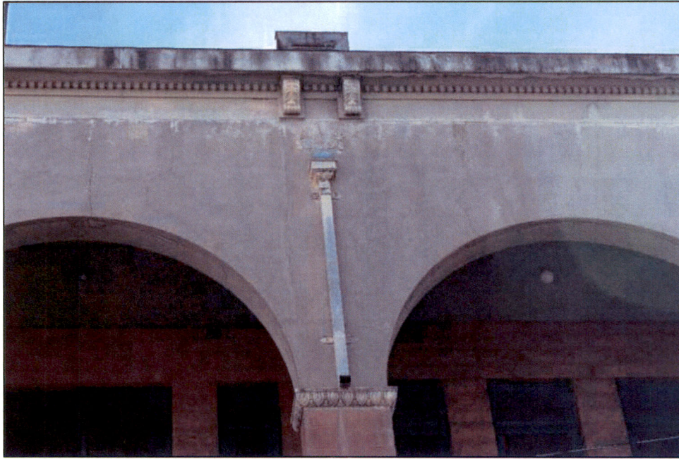
Figure 44. View of entablature, scupper, downspout, and ovolo along north elevation. March 2021.
