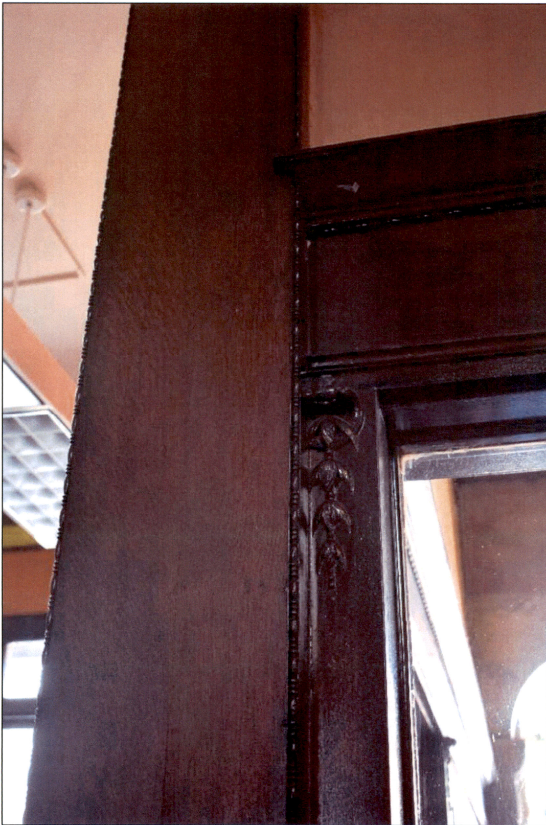
Figure 47. Character-defining molding along second story entry vestibule. Note bead and reel string course and dropped drops of husks, with view looking north. These elements are character-defining and should be preserved or restored. They should not be painted or otherwise altered. March 2021.
