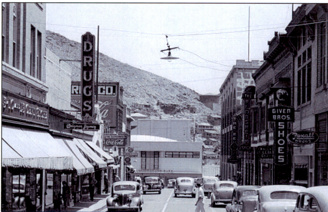
Figure 22. "Wraparound" façade corner visible on right hand side of street. Note cracking in concrete parge coat which likely explains need for later braces. Lee, Russell, photographer. May 1940. Courtesy of Library of Congress.
